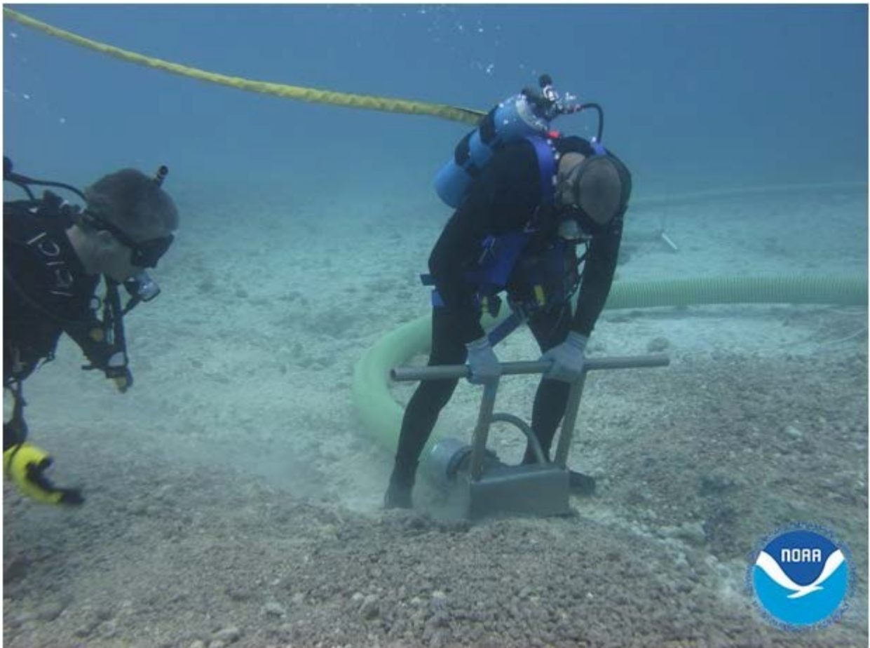
Figure 6. Divers removing rubble from the injury site using a suction hose.
